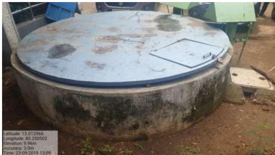
Plate 18: Rain Water Segregation Chamber – D Block
